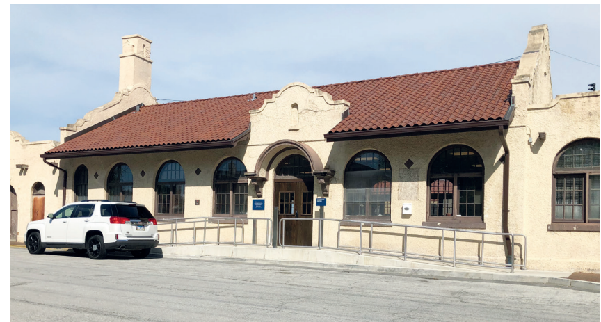
Amtrak made major interior and exterior improvements to its Park Avenue station, including a new tile roof and improvements to make the century old station ADA compliant.
