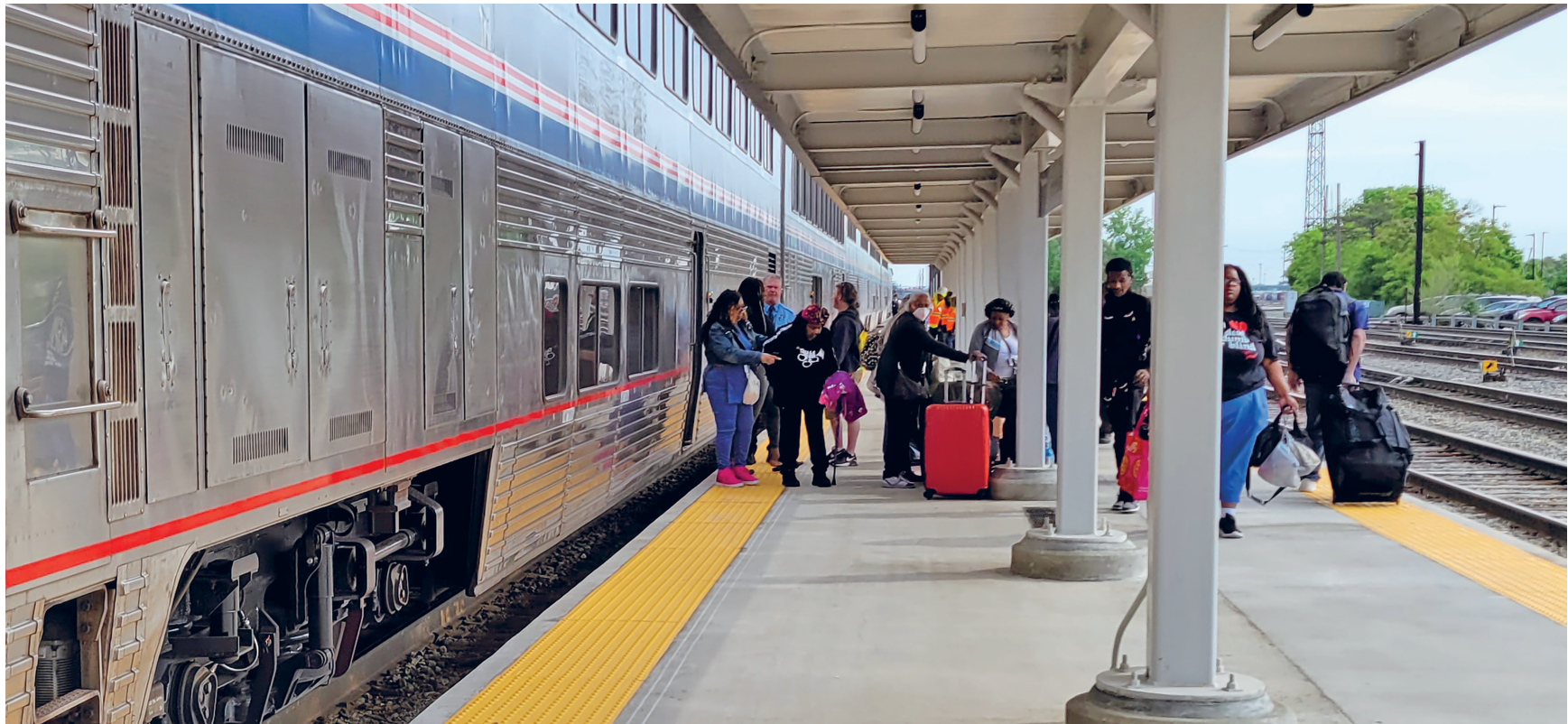
Passengers disembark an Amtrak train on Tuesday, May 24. The new platform was extended, raised to make disembarkment easier, canopied and with improved lighting.
