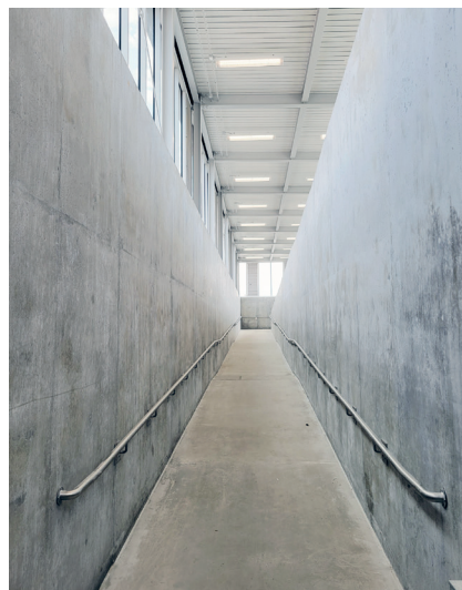
The lower portion of the ramp is finished in this April photo.
